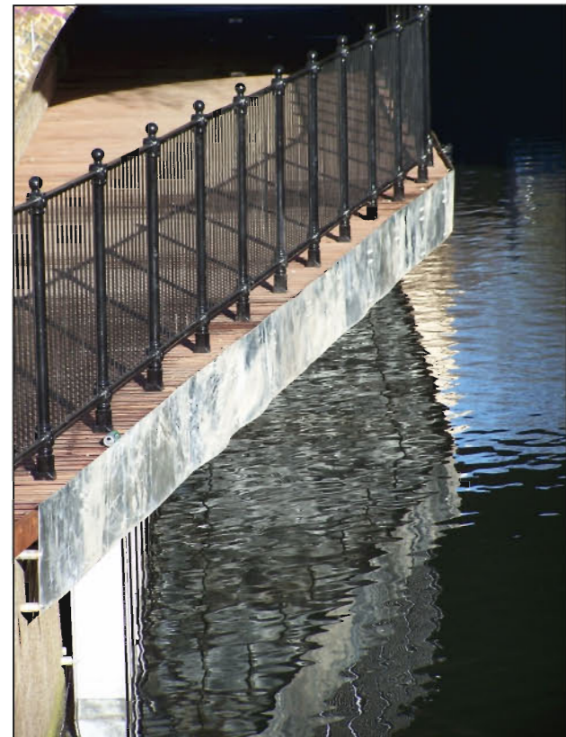
CONTRACTOR'S HANDRAILING DESIGN TO BE SIMILAR TO THAT OF WALKWAY AT MILL POND ROAD
