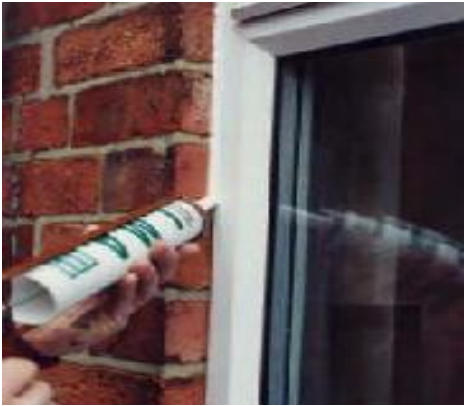
Sealing around a window with mastic
