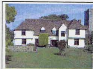
Figure 15- Court Lodge Farmhouse
