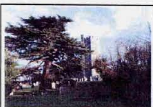
Figure 6- St. Michael's from the north
